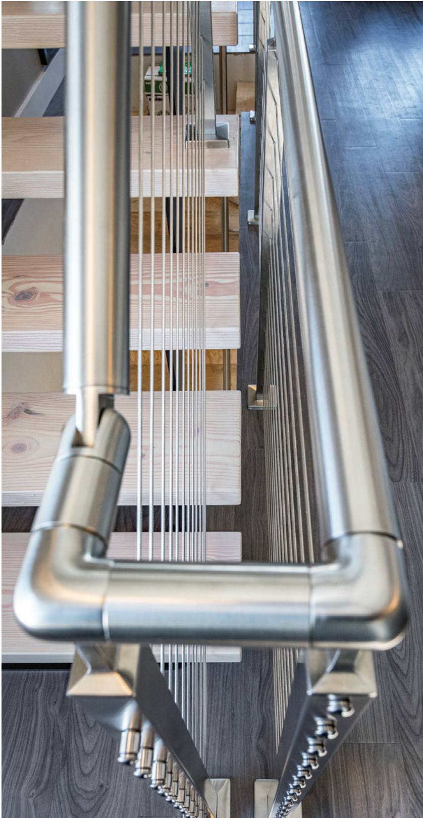
90° round radiused elbow 9231, 0° to 90° round adjustable elbow 9233 and round tube 9010
